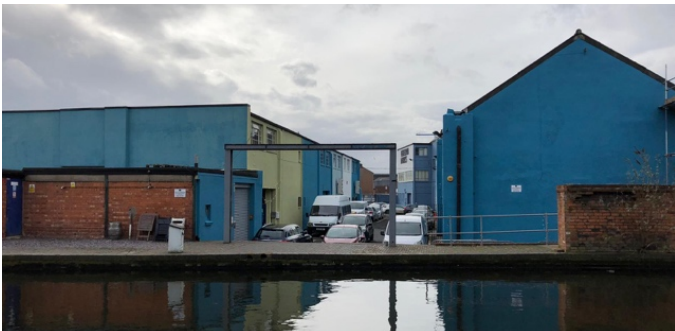
Backside of Minerva Works
