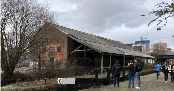
The Banana Warehouse
