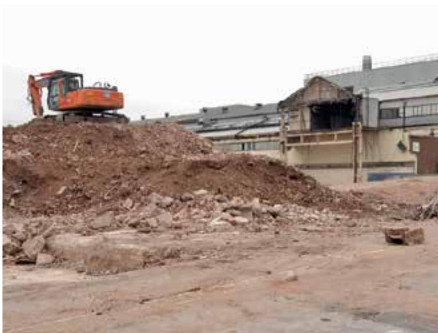
Demolition at Longbridge
