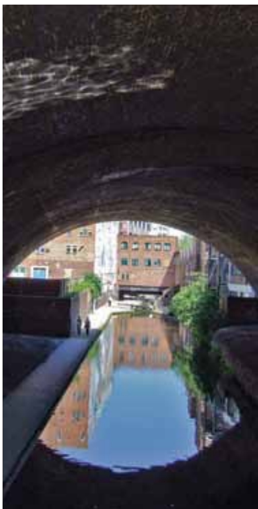
Canal viaduct in the quarter
