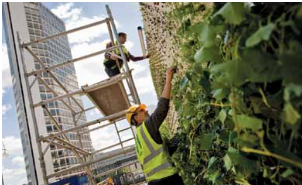
Living wall at the Library of Birmingham construction site
